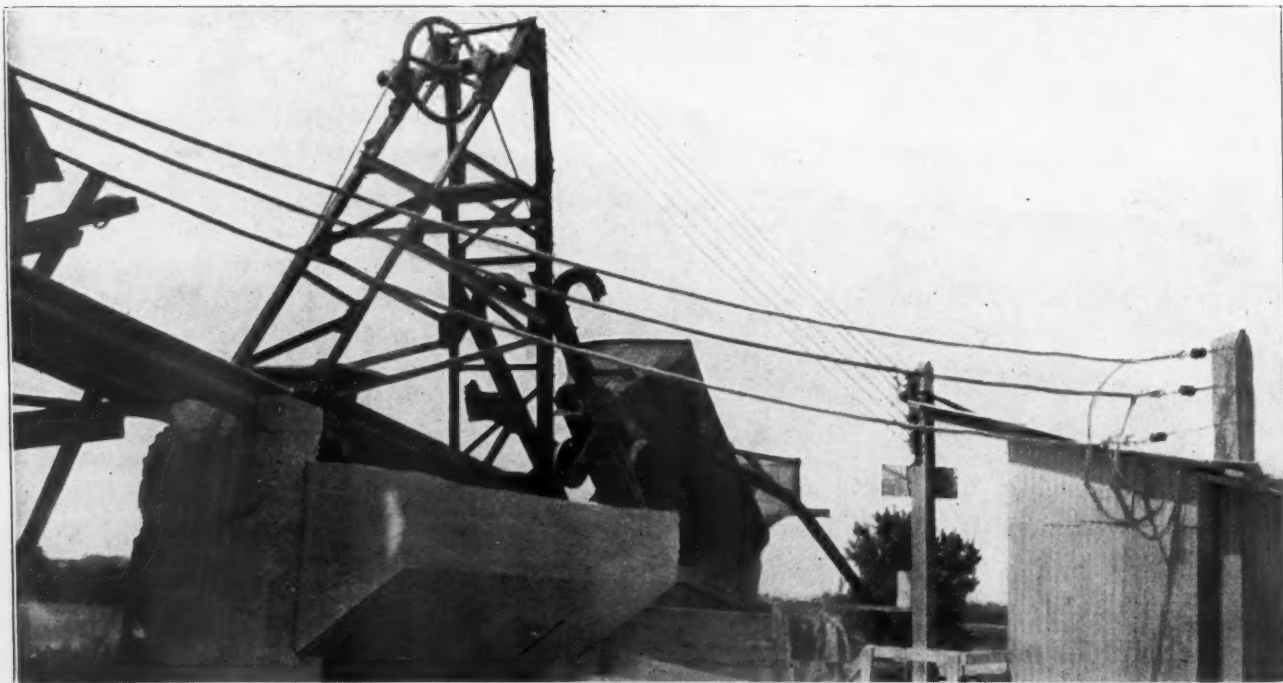
Discharging into Crusher. Note the Concrete Hopper in Left Foreground For Loading Rip Rap
